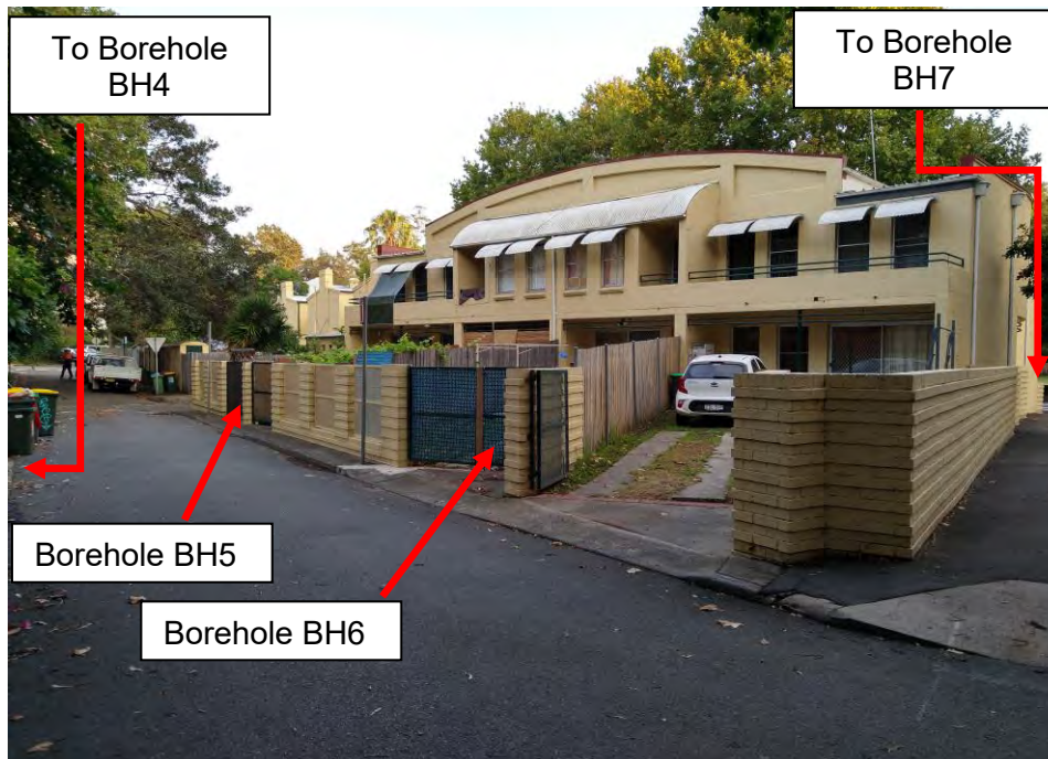
Photograph 10 – View west along Park Lane. The approximate positions of Boreholes BH4 to BH7 are indicated as shown.
