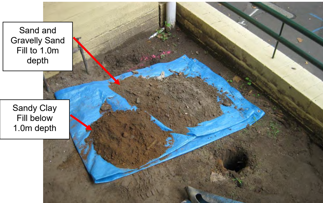
Photograph 14 – View of drilling spoil obtained from Borehole BH7.
