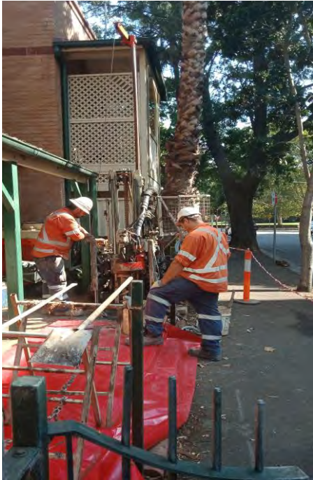
Photograph 6 – View north along Cowper Street at Borehole BH2.
